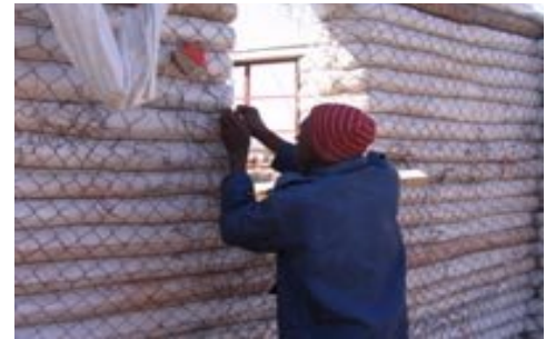
Above: Fastening wire mesh as a base for concrete stucco.
