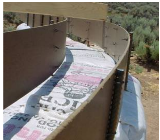
Above: Rebar serve as braces for the bond beam form.
